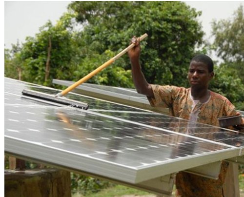
(b) Cleaning solar panel
