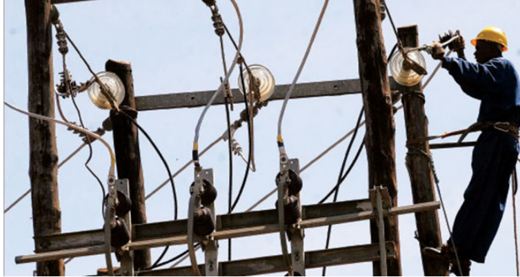
Fig. 4.6: Higher capacity transmission lines being set up
